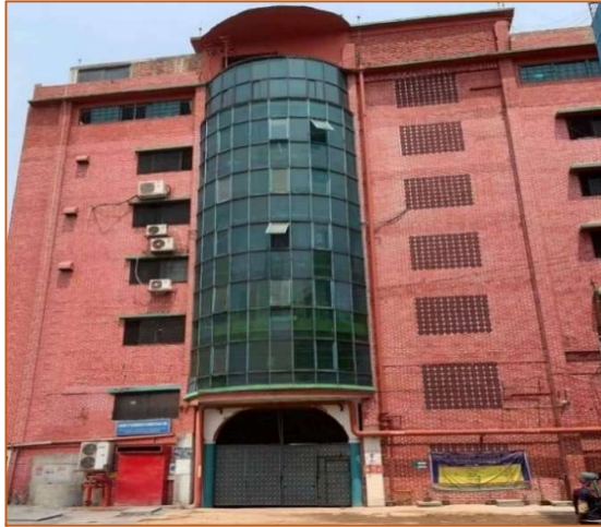
Factory Front View
